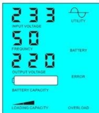
Battery dead, utility supply power
