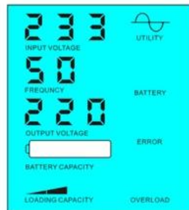
Battery unavailable, utility supply power
