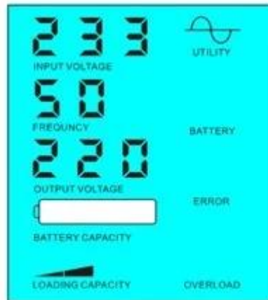
Battery dead, utility supply power
