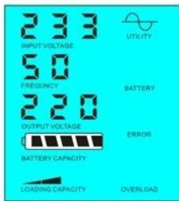
Utility supply power and charge battery
