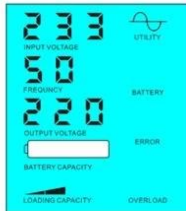
Battery dead, utility supply power
