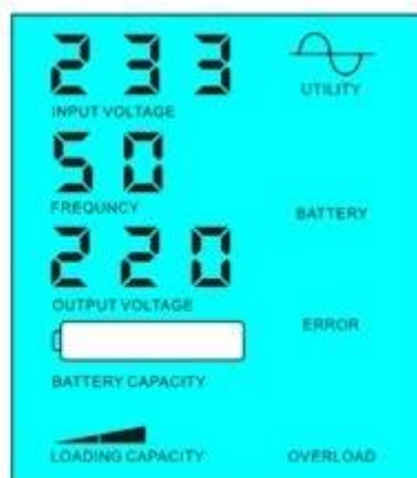
Battery dead, utility supply power
